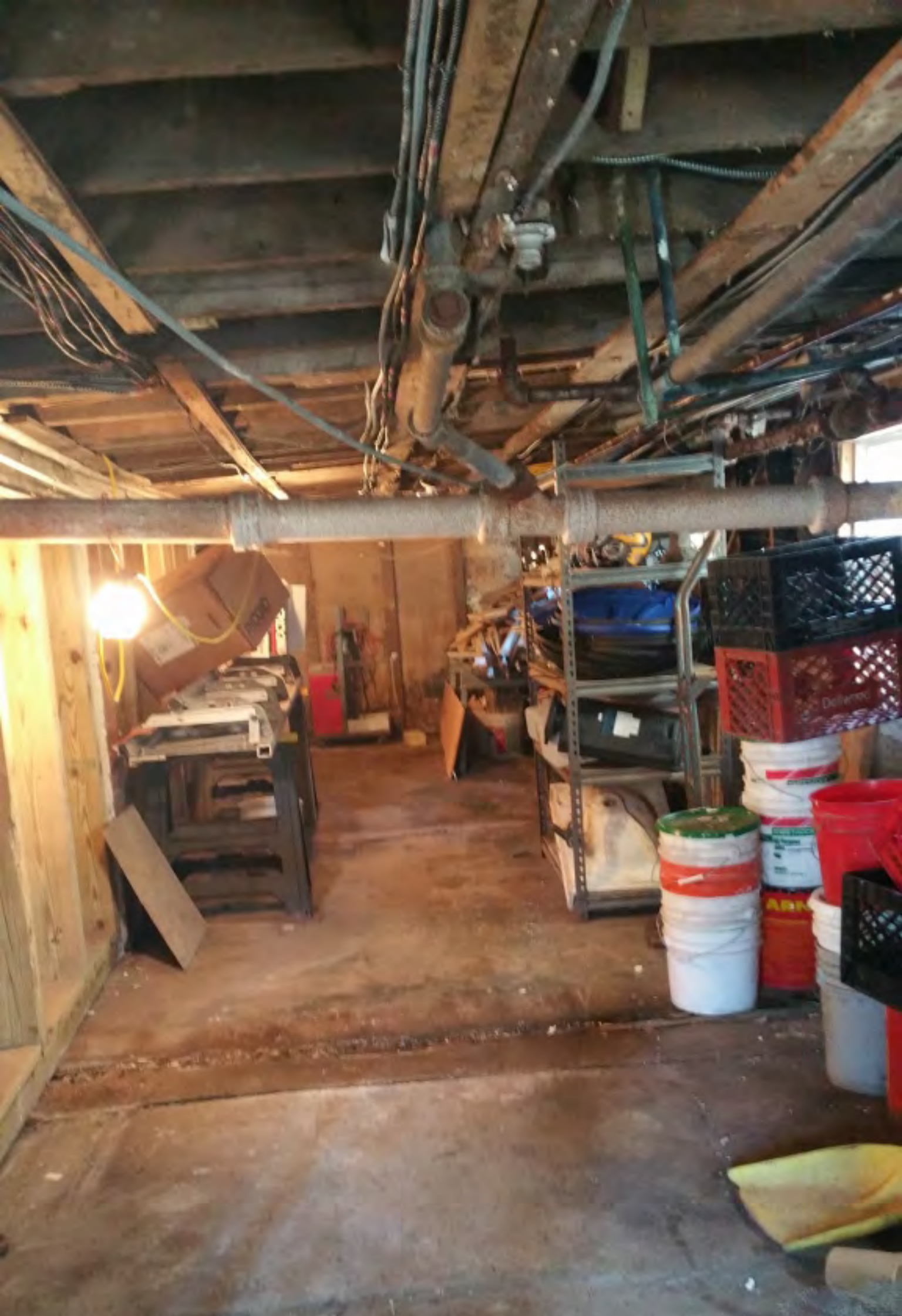
BASEMENT - FRONT BUILDING
